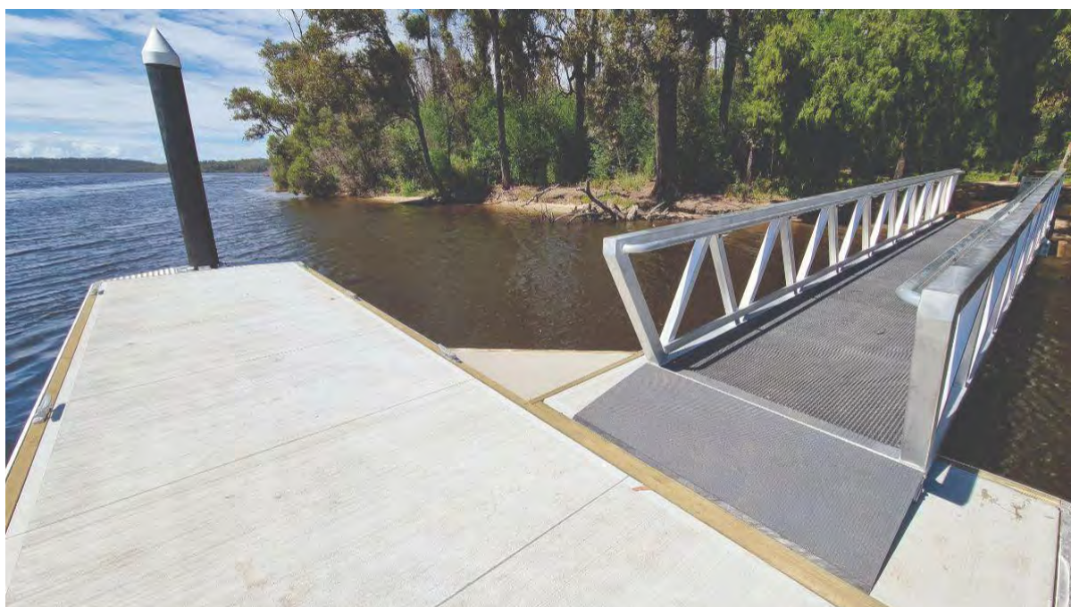
Figure 26: Floating pontoon jetty at Genoa River. Photo: Parks Victoria
